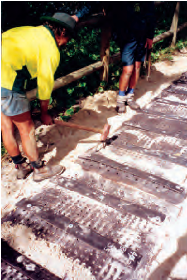
Photo # 6: Shows the use of inverted U pegs, each about 700 mm long and 16 mm thick (deformed bar is best) driven into the sand at various points along the track. It is best to lay holeybelt on a hot day, and stretch it a bit before driving in the pegs. Use a 4 WD or tractor to stretch it.
