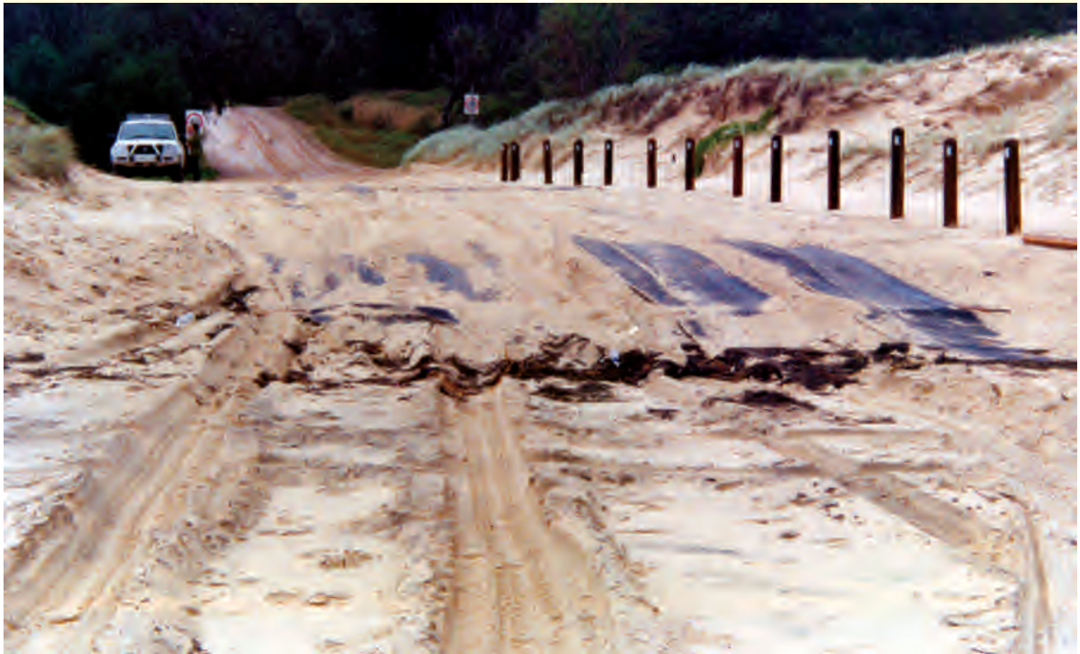
Photo #5. Access to beaches on the intertidal zone can be tricky, even for experienced 4WD users. Many a vehicle has been stranded at this point to suffer various degrees of inundation with salt water when the tide rises. Here Holeybelt only about 40 metres long bridges the tricky portion, allowing secure escape from the beach, and also minimising disturbance of the sand.
