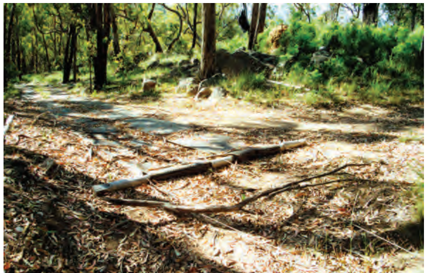
Photo # 7: Shows Holeybelt fixed into sand with a hardwood bearer and marine ply gusset plate. This detail allows the Holeybelt to be easily removed and reinstalled in case it is disturbed by a tidal surge.
