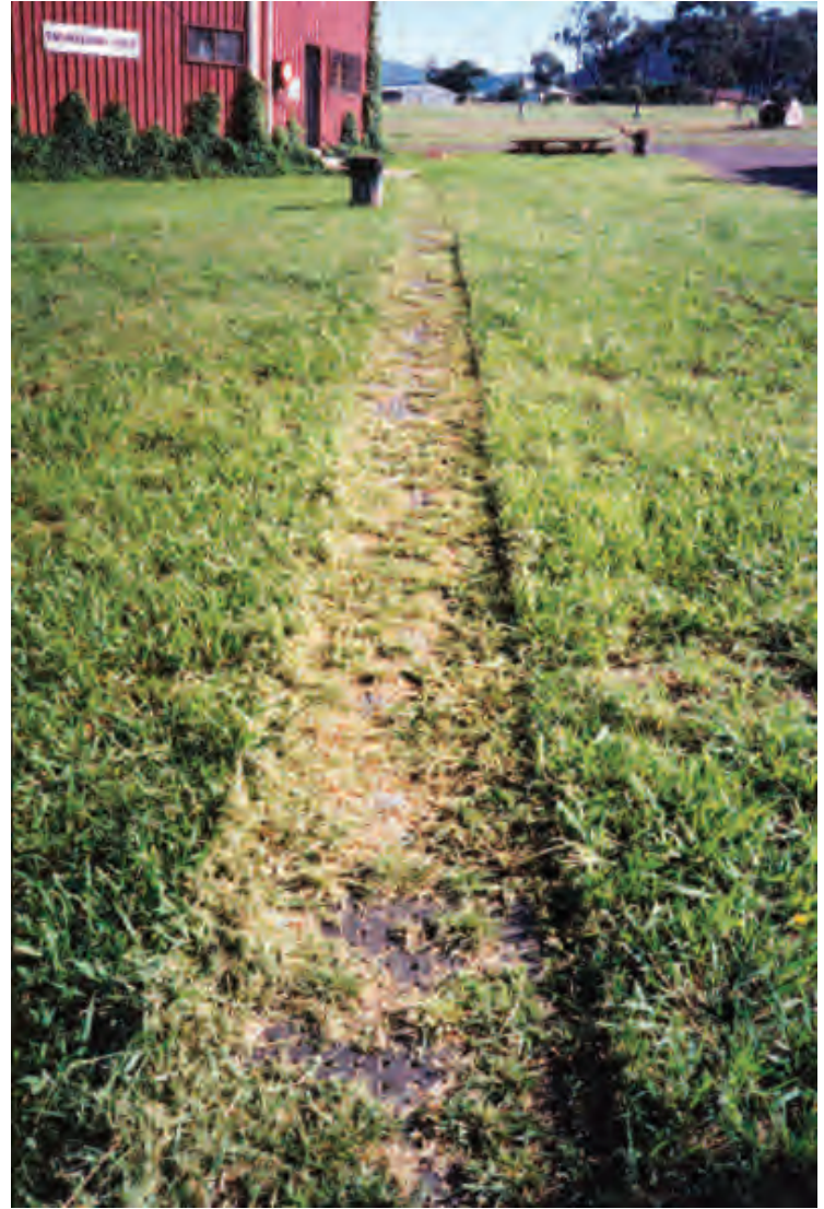
Photo #3. After 12 months the holeybelt virtually disappears and sinks into the ground, so that mowers can pass clear over it. This walkway is only 400 mm wide, yet is adequate for a lot of pedestrian traffic.
