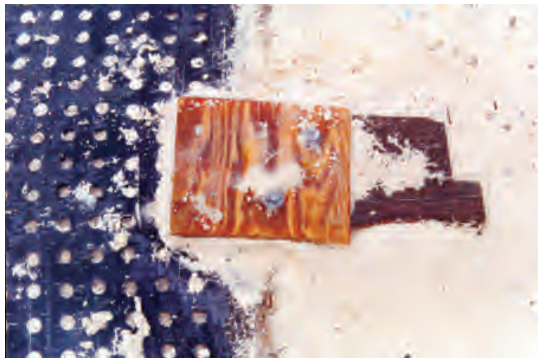
Photo # 7: Shows Holeybelt fixed into sand with a hardwood bearer and marine ply gusset plate. This detail allows the Holeybelt to be easily removed and reinstalled in case it is disturbed by a tidal surge.
