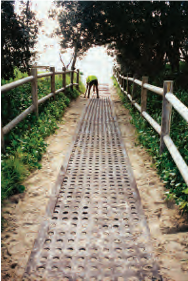
Photo #2. Holeybelt walkway installed by Coastcare NSW provides an attractive and softer alternative to board and chain.
